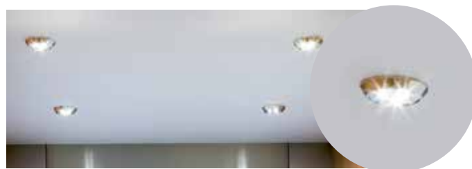
Ceiling with LED spots
