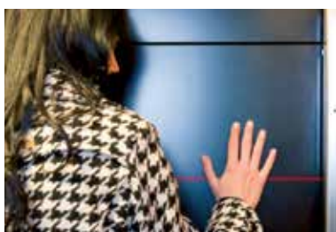
2D optically-activated emergency lift car stop mechanism
