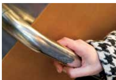
Stainless steel handrails
